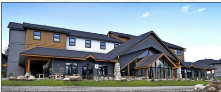
Photo courtesy of Horizon North Modular Solutions.
